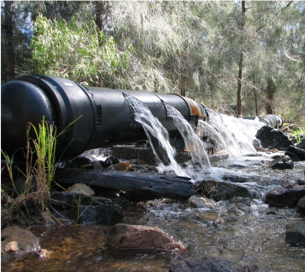
Figure 1 – SGWTF Discharge Location
