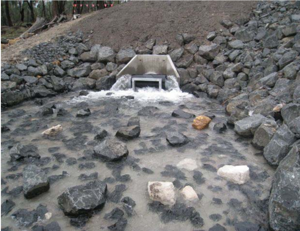
Figure 1 - TWTF Discharge Location
