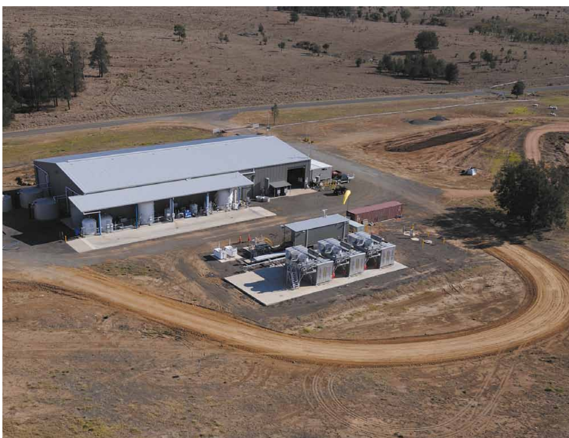
Australia Pacific LNG's operating water treatment facility at Spring Gully, near Roma
