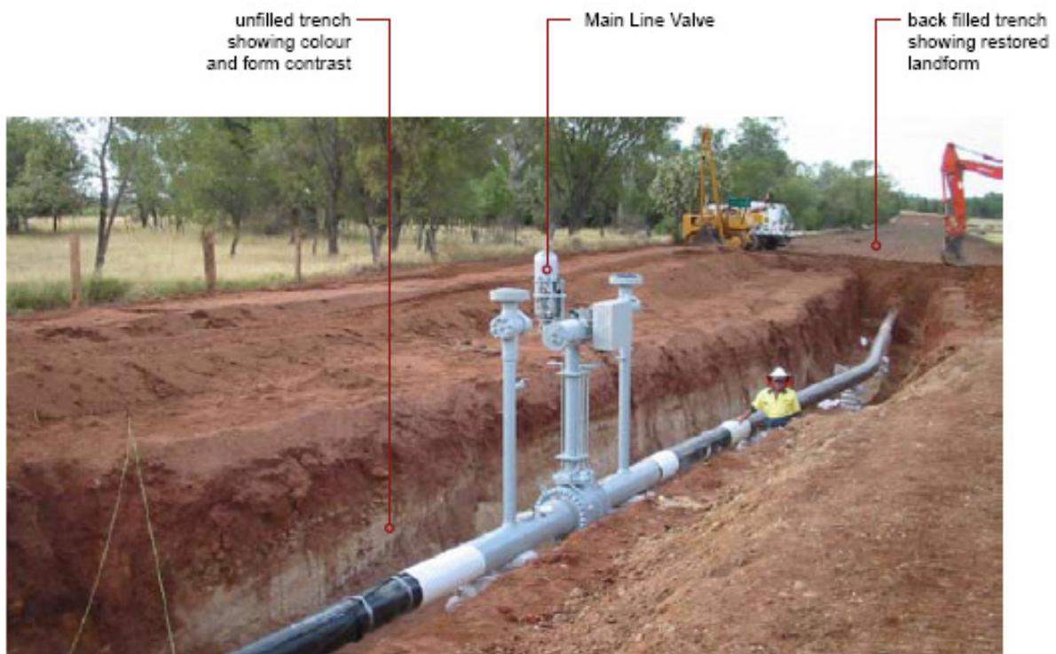
Figure 7.3 Typical pipeline construction – mainline valve
