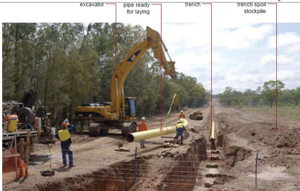
Figure 7.2 Typical pipeline construction – lowering pipes
