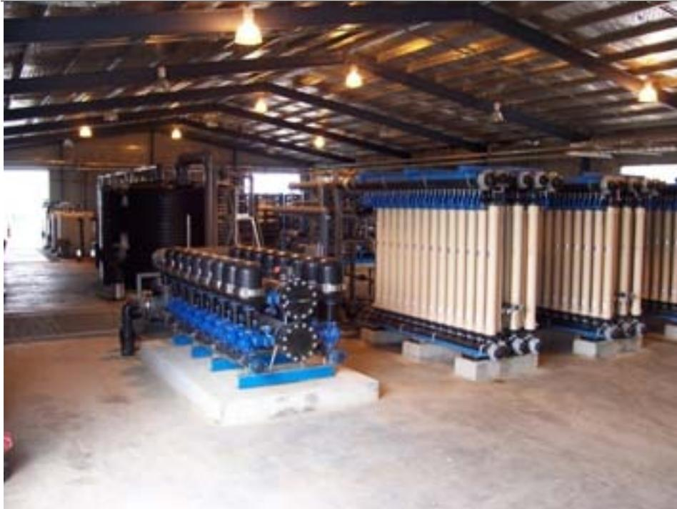
**Plate 6.2 Membrane filtration system at Spring Gully WTF**
