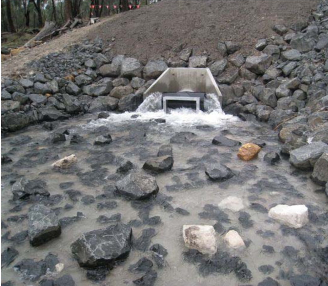
Figure 1 - TWTf Discharge Location
